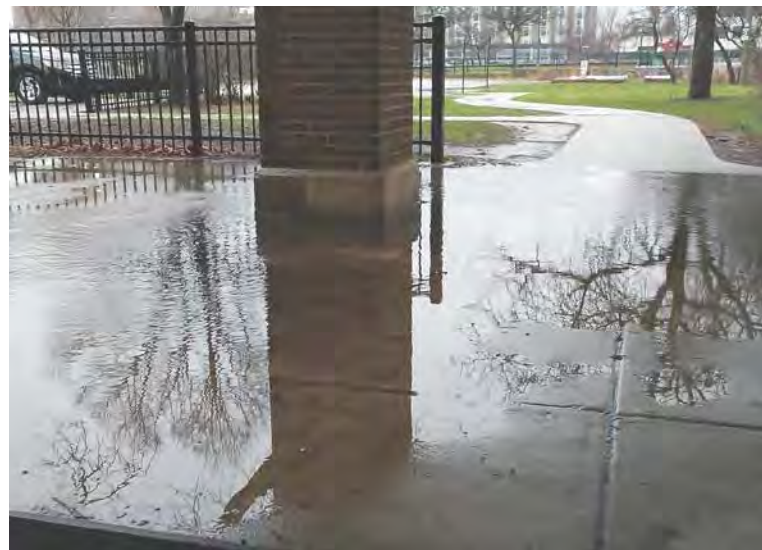
EXISTING FLOODED BUILDING ENTRY
