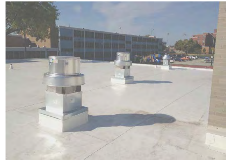
POTENTIAL ROOF IMPROVEMENTS
