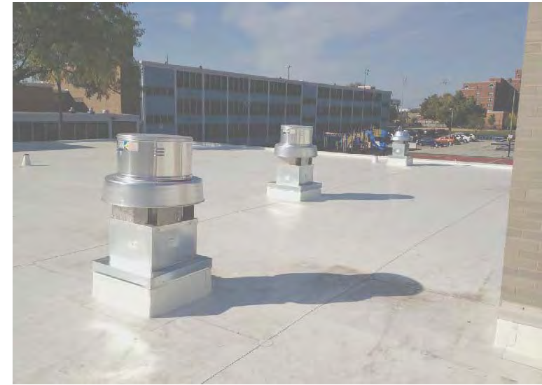
POTENTIAL ROOF IMPROVEMENTS
